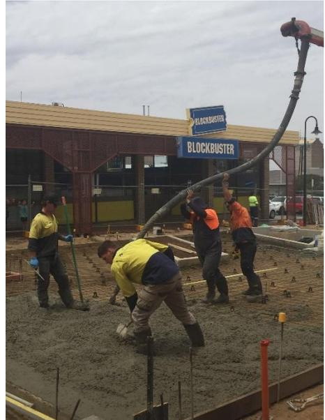
A concrete pavement being poured in Zone 2.
