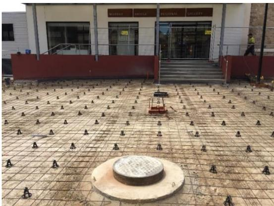
Steel reinforcement ready for the concrete pavement outside the Art Gallery
