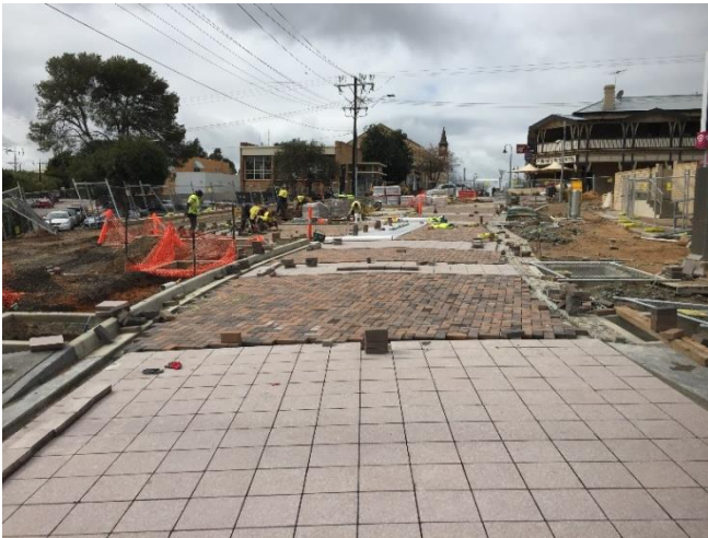
New block paving underway at the Northern end of Sixth Street
