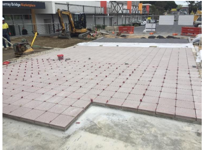
New block paving underway on South Terrace
