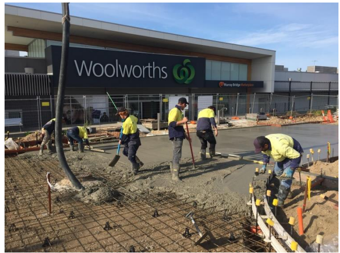
New concrete pavement being poured on South Terrace
