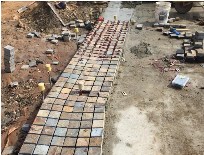
Feature paving being laid for the new dish drains
