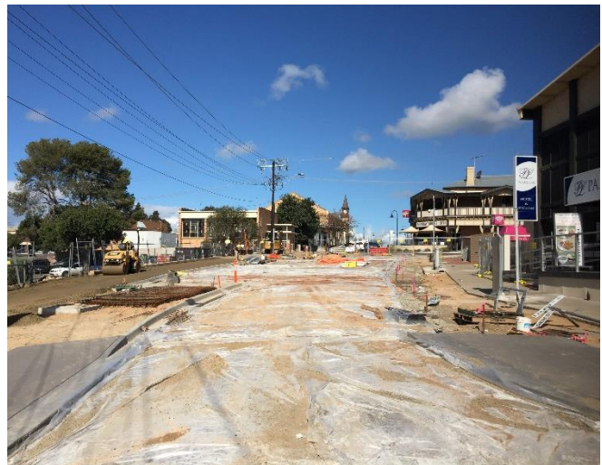
New concrete pavements are covered in plastic while curing
