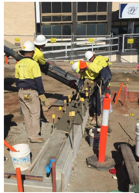
Kerb installation is underway in Zone 5
