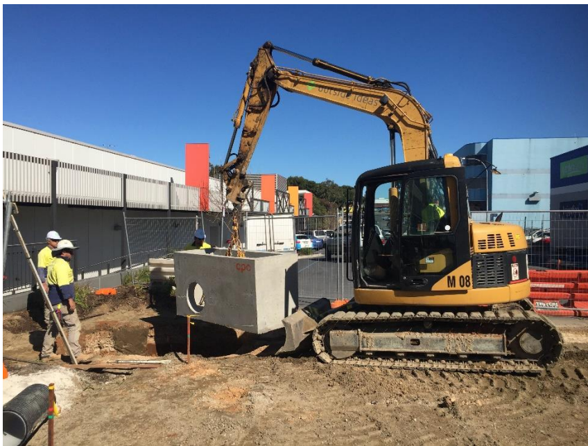
A new drainage pit is installed in Zone 1
