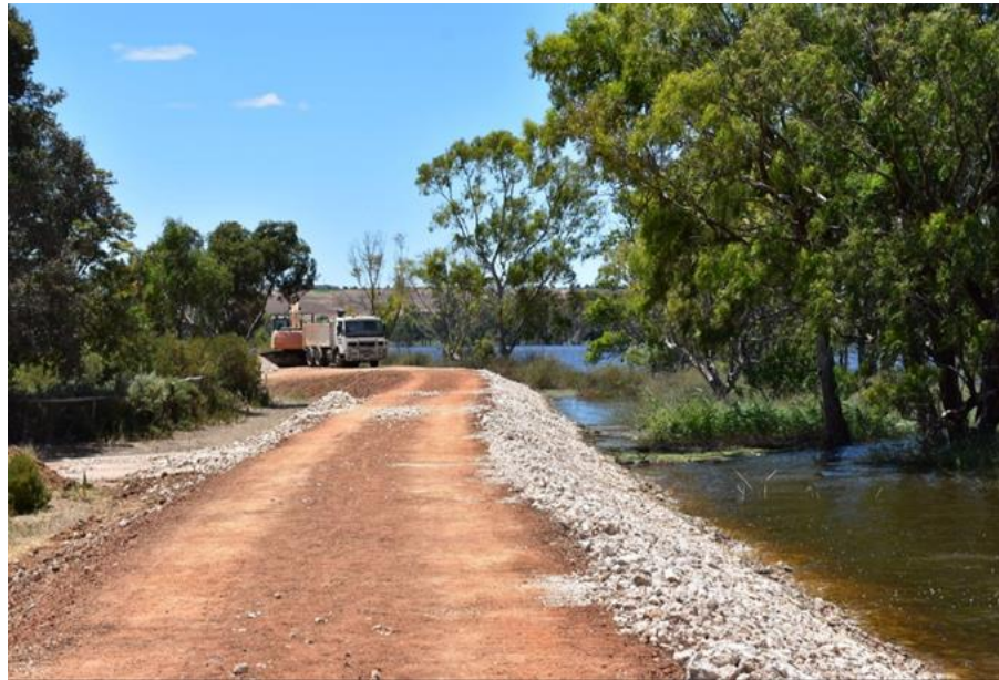
Mypolonga Levee – 5 January 2023
