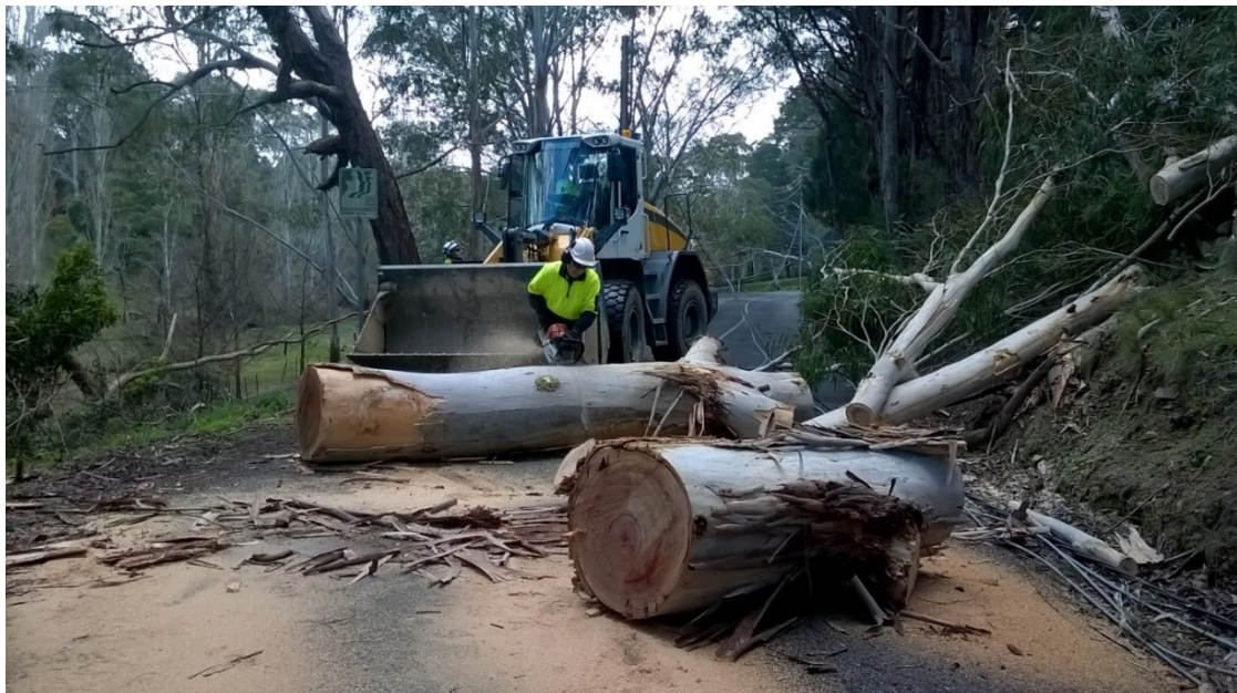
Figure 2: Workers clearing fallen tree off of road after a natural disaster
