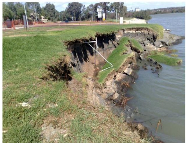
Figure 8 Riverbank slumping on the River Murray caused by prolonged low river levels during the Millennium Drought
