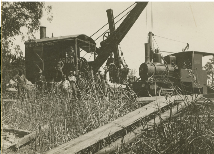
Steam navy & locomotive used for construction work, 1915. PRG-1258-59-210
