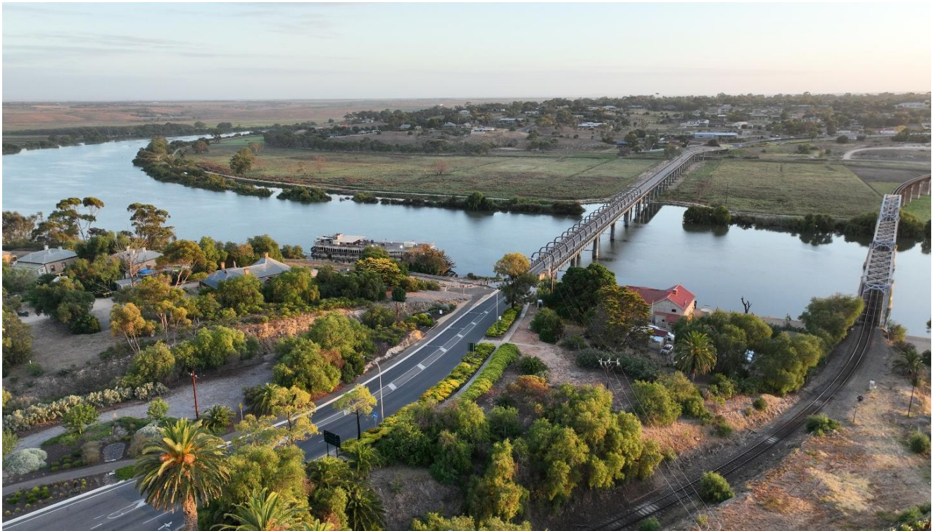
Image credit: Drone photo of the Murray Bridge and Railway Bridge.
