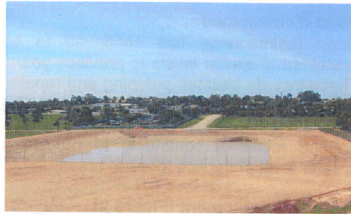
Figure 7 – Greenlands Drive Stormwater Pond
