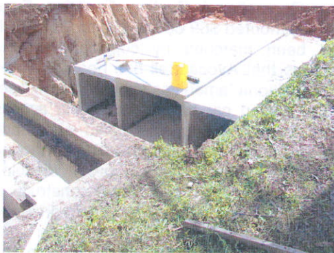
Figure 6 – Culverts under Adelaide Road
