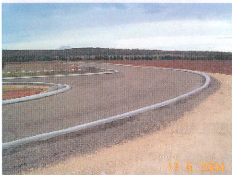
Figure 17 – Bremer Road Cemetery – new road and kerbing
