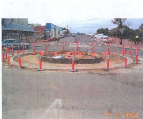
Figure 4 – Roundabout under construction
