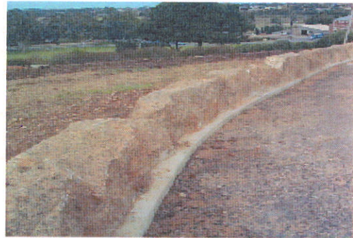
Figure 13 – Wharf Hill – recycled granite
